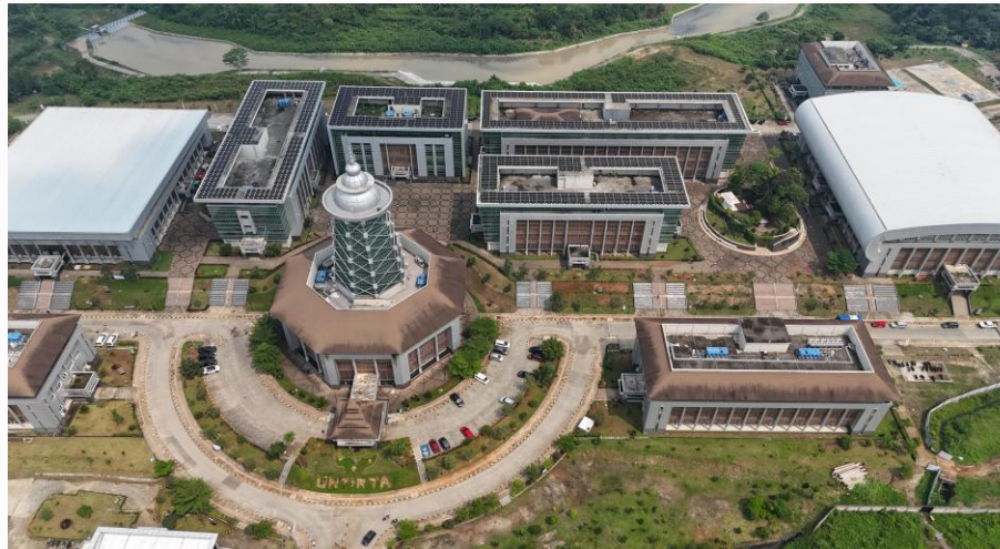
Rooftop Solar Panel Universitas Sultan Ageng Tirtayasa
